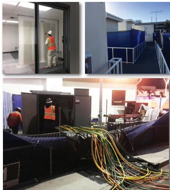
Electricians complete extensive tie-in to permanent power for the trailer complex.
